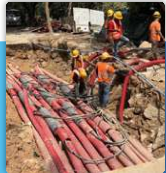
33kV Power Cabling Works
