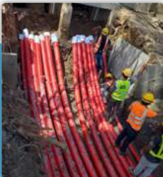
11kV Power Cabling Works
